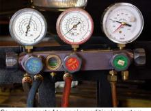
Gauges connected to an air conditioning system
